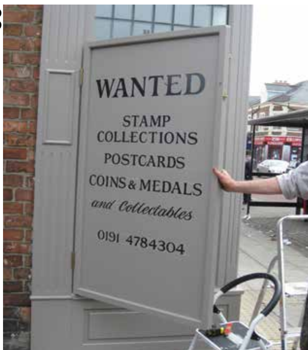
The Stamp Shop features a side hung A-board advert which forms part of the restored shop-front.
